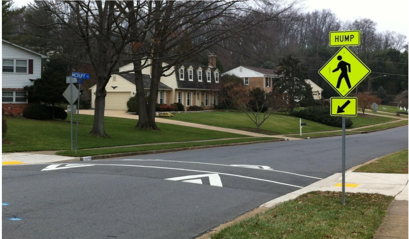
Figure 9.1 - Raised Crosswalk
