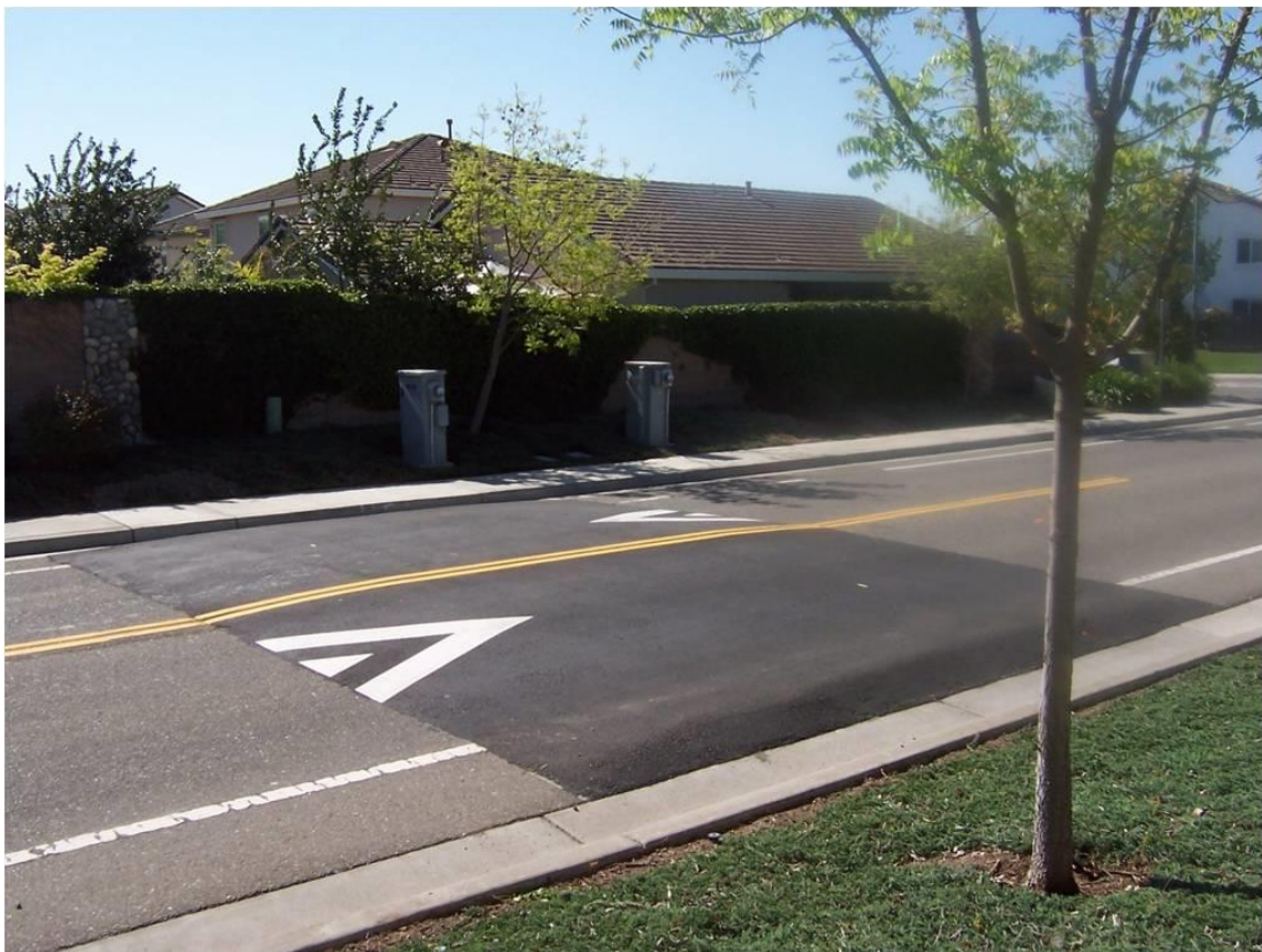
Figure 7.1 - Speed Table
