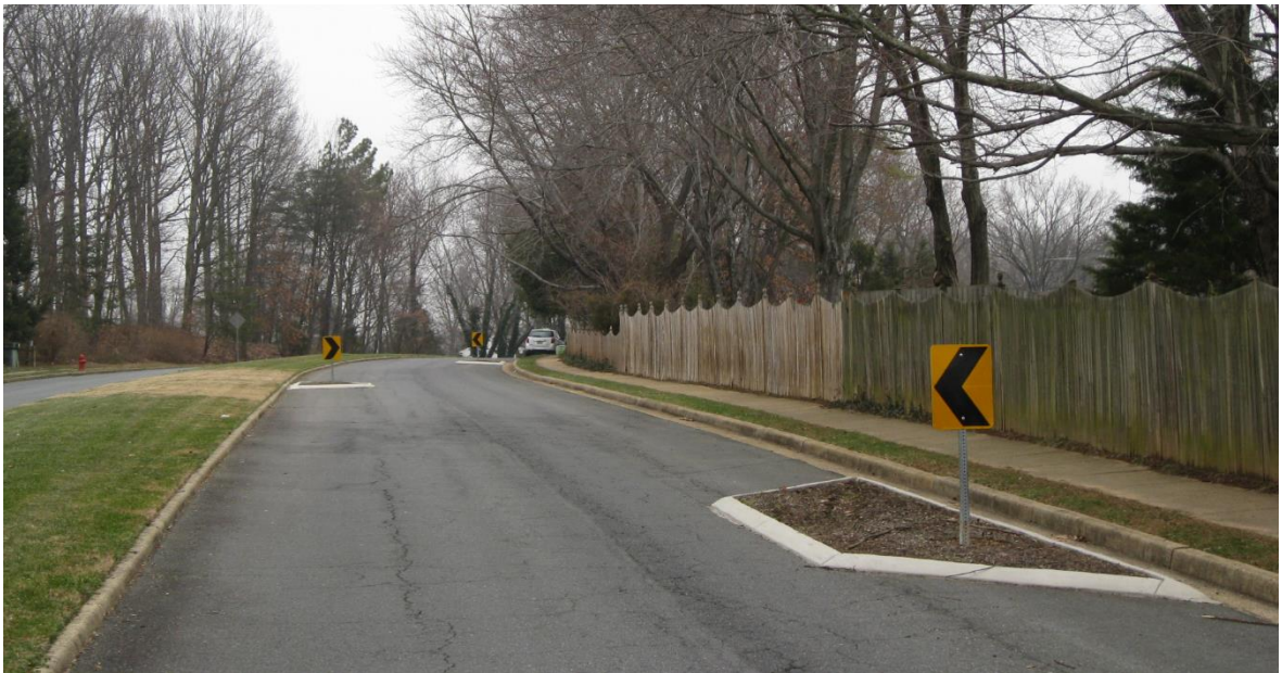
Figure 12.1 – Chicane (Single lane, One-way travel)
