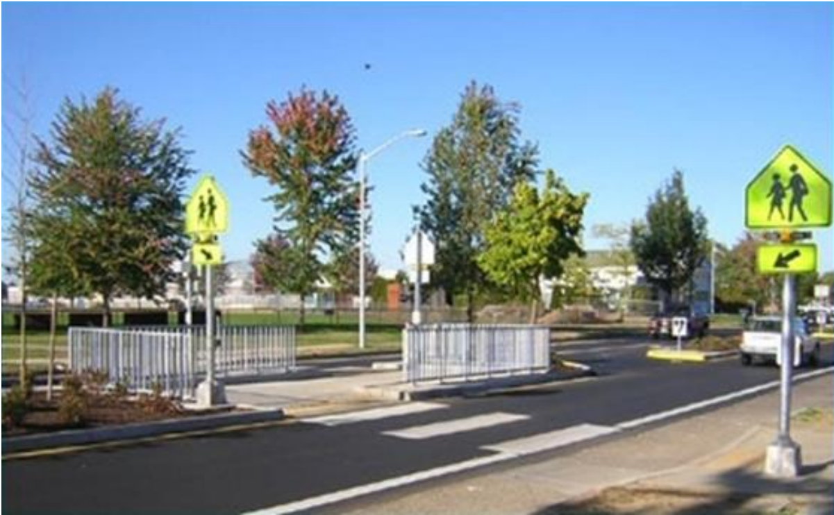
Figure 11.2 - Crosswalk Refuge –Offset “Z”-option
