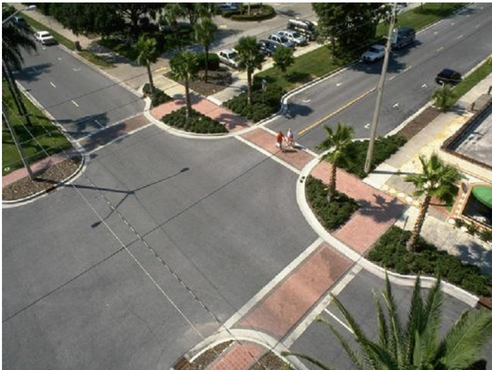
Figure 14.1 –Curb Extension (Neckdown)
