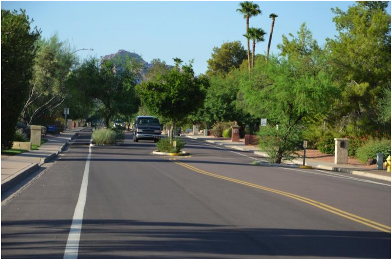
Figure 12.3 – Chicane (Two-way travel)
