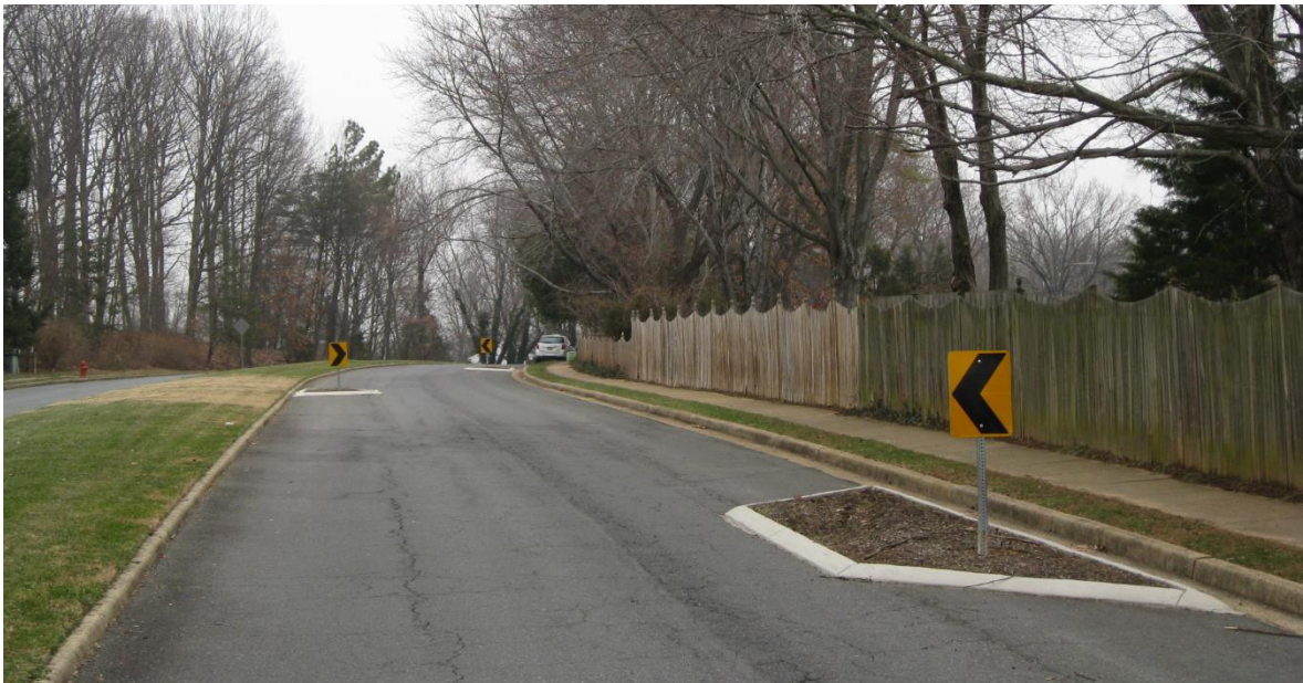
Figure 12.1 – Chicane (Single lane, One-way travel)
