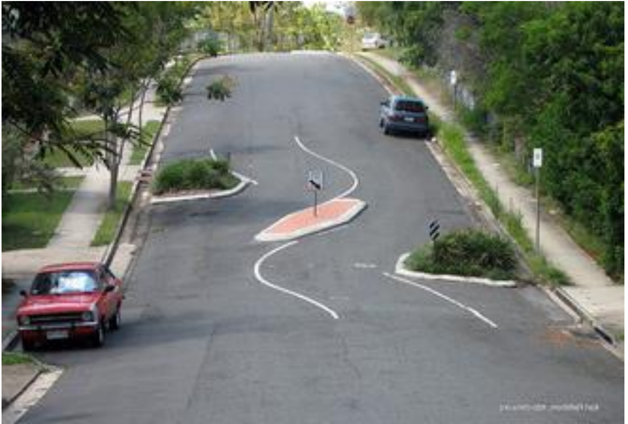
Figure 12.2 – Chicane (Two-way travel)
