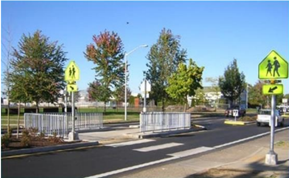
Figure 11.2 - Crosswalk Refuge –Offset “Z”-option
