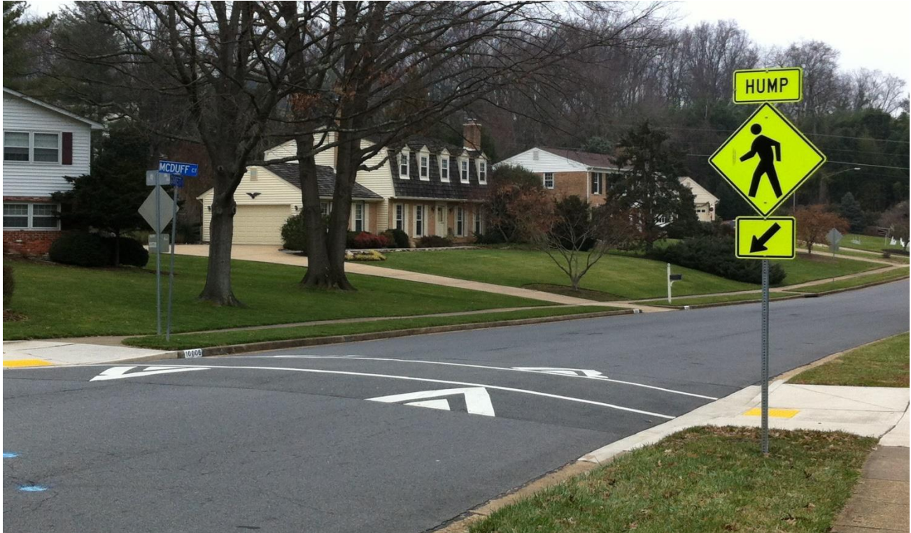
Figure 9.1 - Raised Crosswalk
