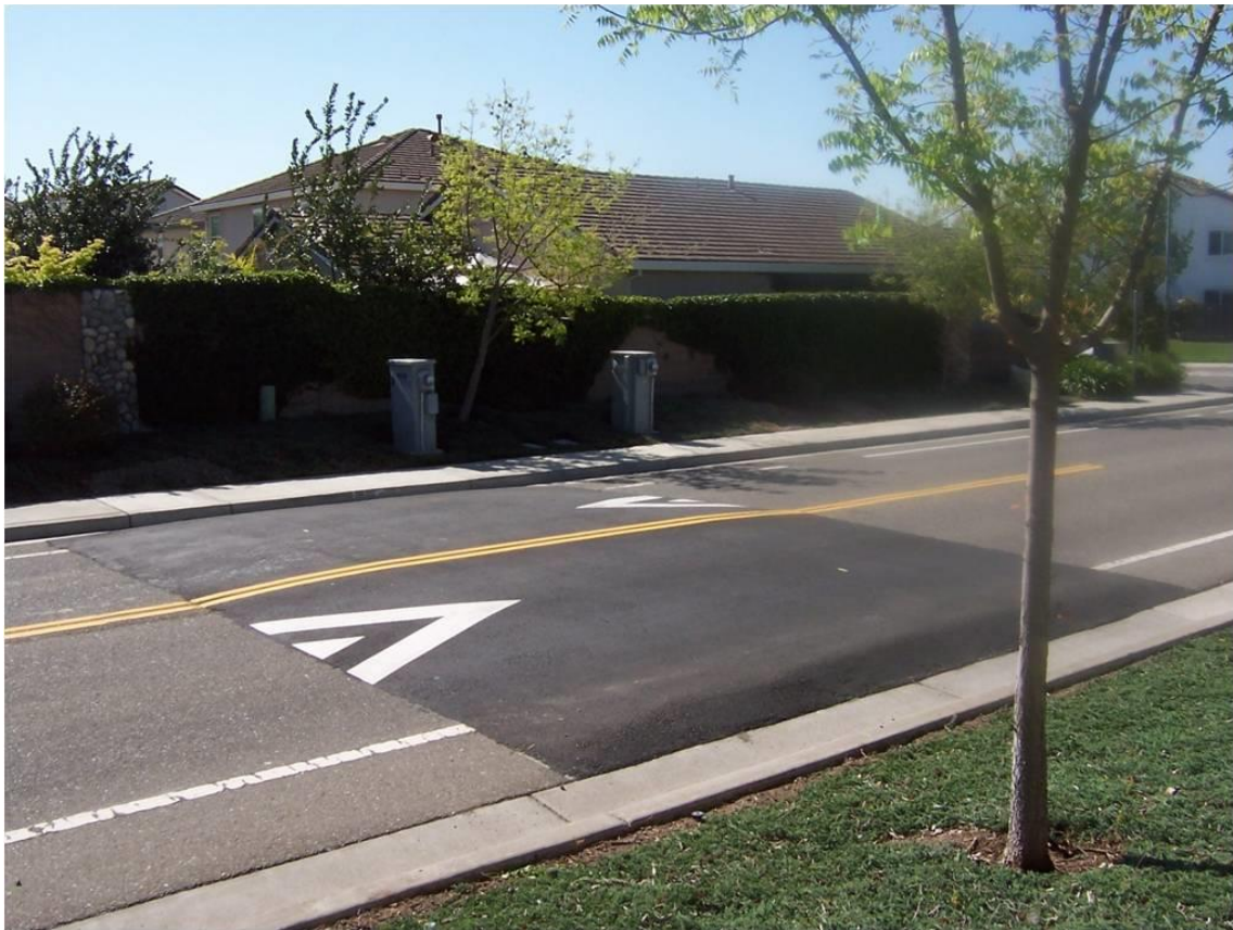
Figure 7.1 - Speed Table
