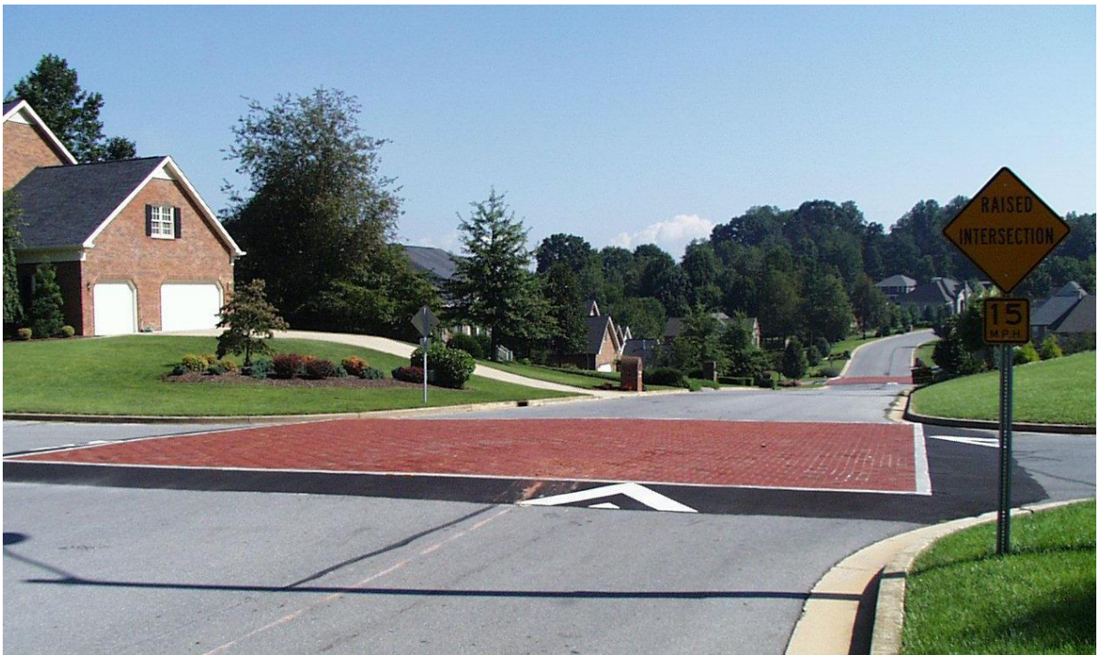
Figure 8.1 – Raised Intersection
