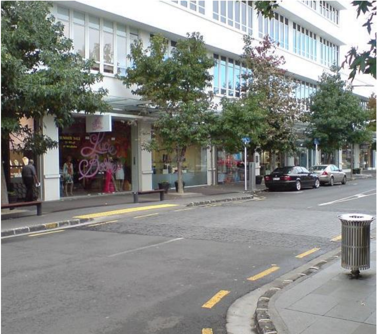
Figure 7.2 – Speed Table
