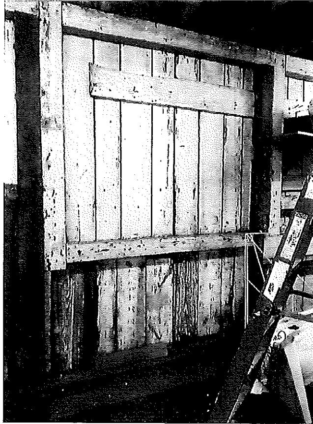
Figure 5 - West wall framing example below floor.
