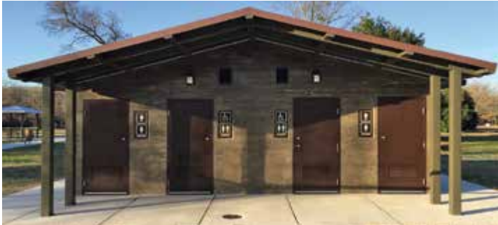
Flush restroom with custom simulated wood texture and awning
