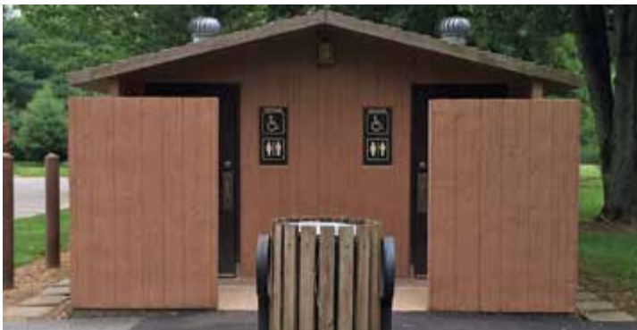
Double vault restroom with privacy screen
