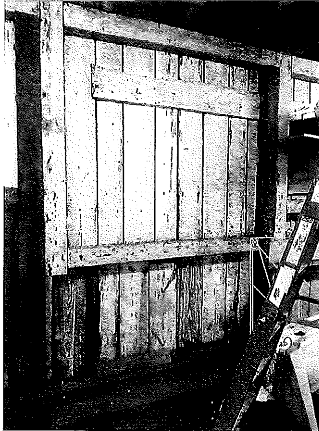
Figure 5 - West wall framing example below floor.
