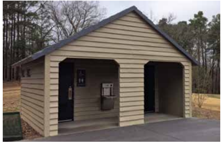
Flush restroom with custom golf cart shelter
