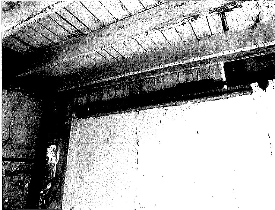
Figure 3 - View of floor framing.
