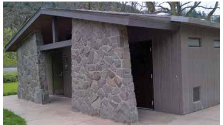
Flush restroom with custom covered entry
