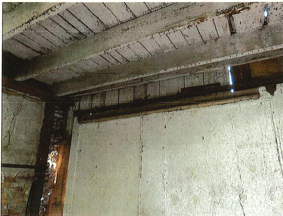
Figure 3 - View of floor framing.
