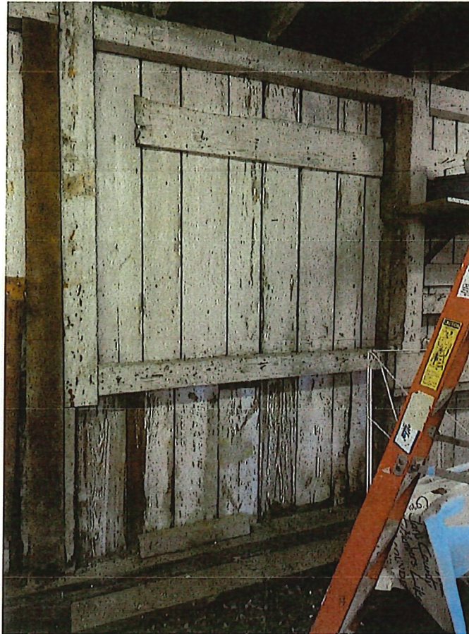
Figure 5 - West wall framing example below floor.
