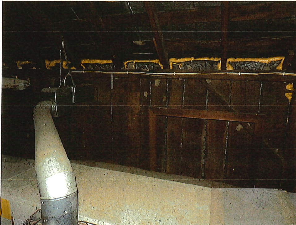
Figure 4 - Typical west wall framing above floor level.
