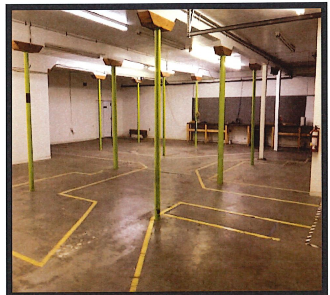
2,600 SF Warehouse 12 foot Ceiling
